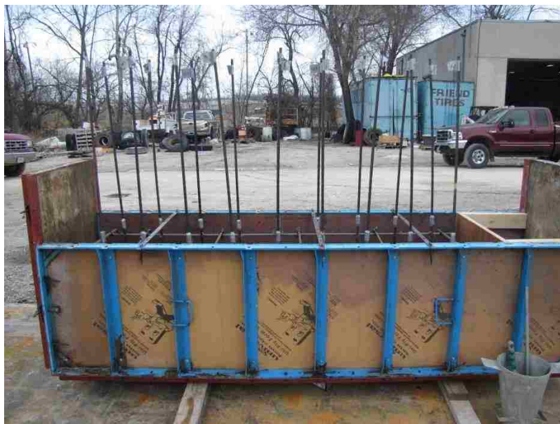
Figure 3.22 – LBPT Specimen Before Casting
