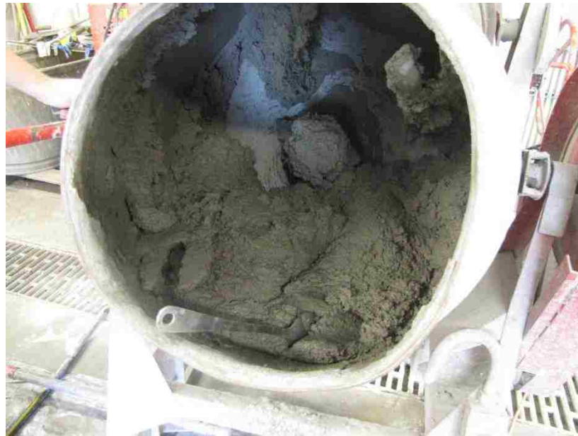
Figure 3.7 – Mortar Mix in Drum Mixer
