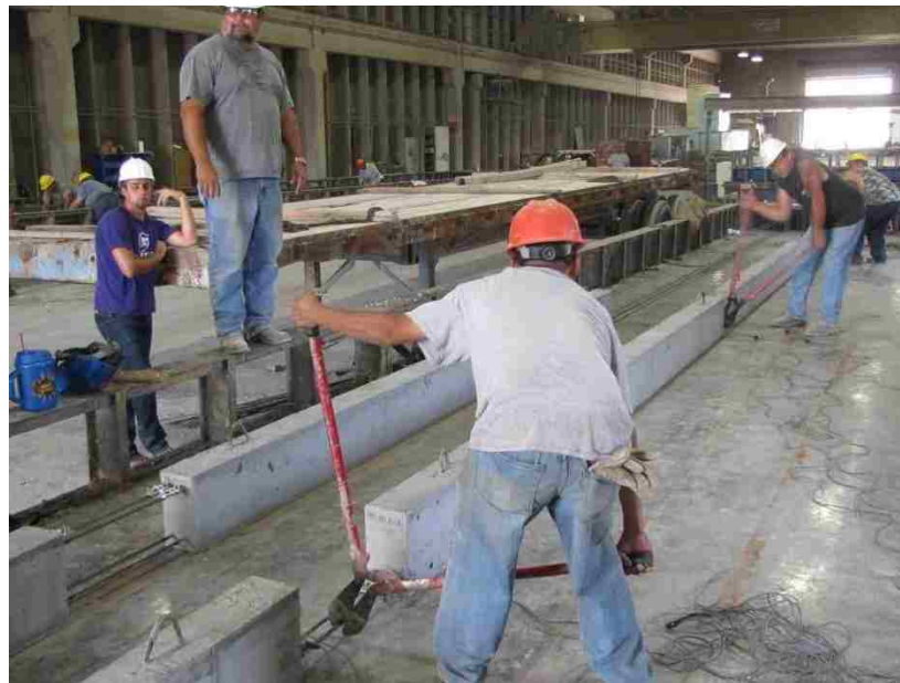
Figure 4.10 – Bolt Cutting Strands at Release
